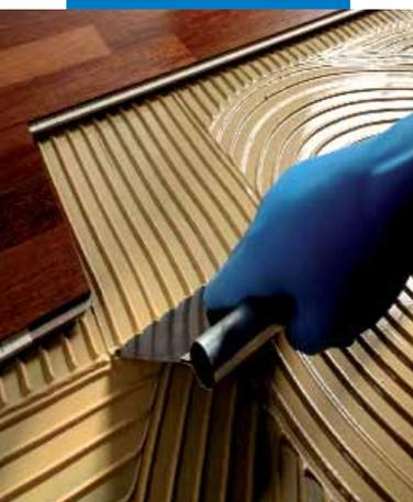
Laying large format of pre-finished parquet with Ultrabond Eco S955 1K
