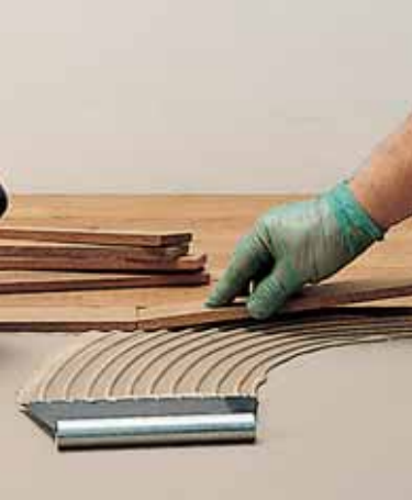
Installing MUHUUH wood strips
