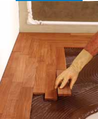
Installing a 14 mm Teak plank
