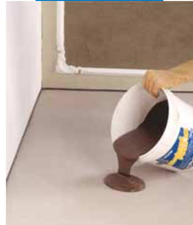
Pouring the adhesive onto the screed
