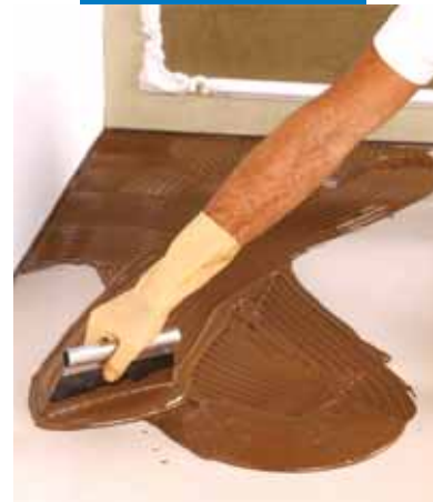
Applying the adhesive
