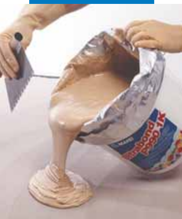
Pouring the adhesive on a screed
