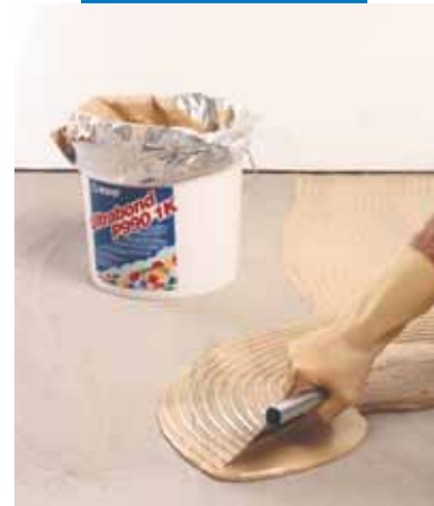
Spreading the adhesive
