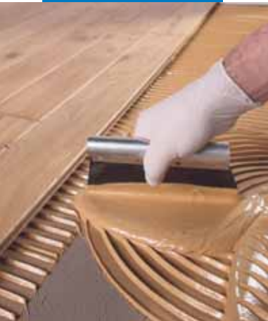
Spreading Ultrabond P990 1K
