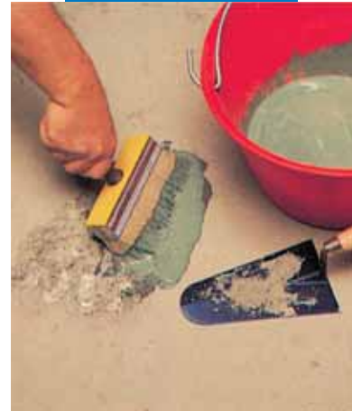
Floor patching: application of slurry
