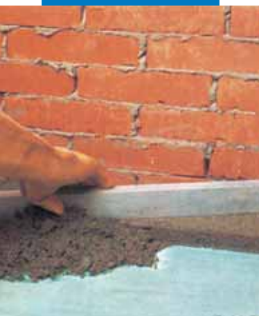
Application of cementitious screed with Planicrete admix
