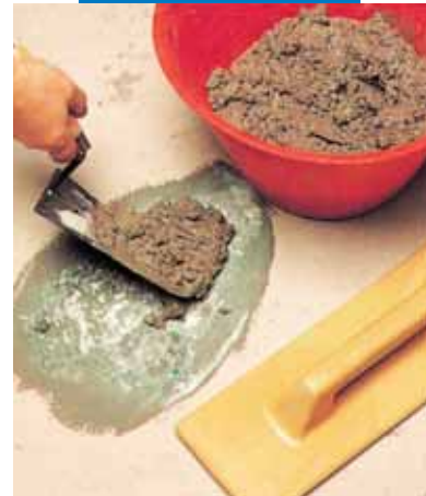
Floor patching: application of mortar
