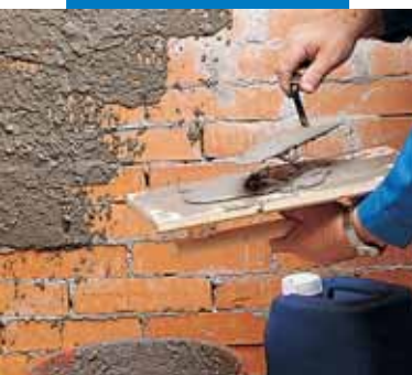
Base-keying mortar layer with Planicrete admix
