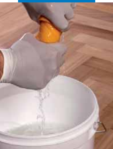
Diluting Ultracoat Universal Cleaner into clean water: dip the cloth into water and squeeze it thoroughly
