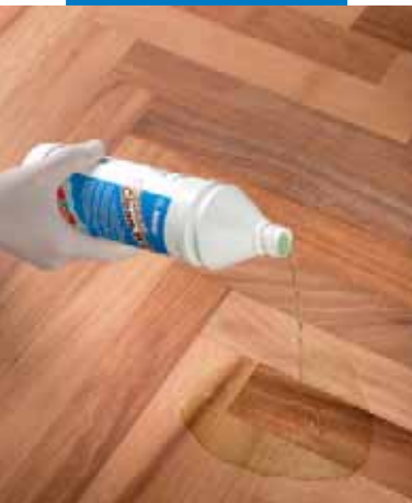
Example of Ultracoat Clean WPM used undiluted: apply a small quantity of product to the floor
