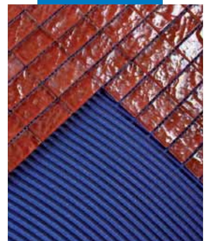
The following day, grouting with Kerapoxy Design in the same colour and the same application procedure previously shown
