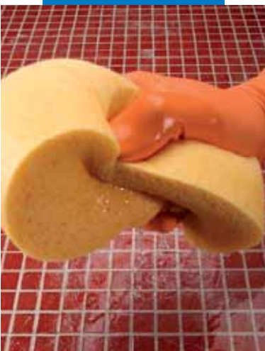
Wetting the surface of the grout before cleaning
