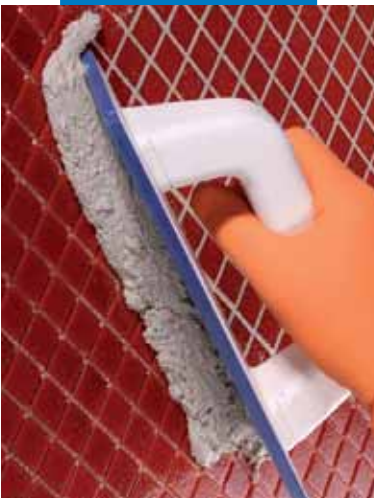
Application of Kerapoxy Design with a hard rubber grout float
