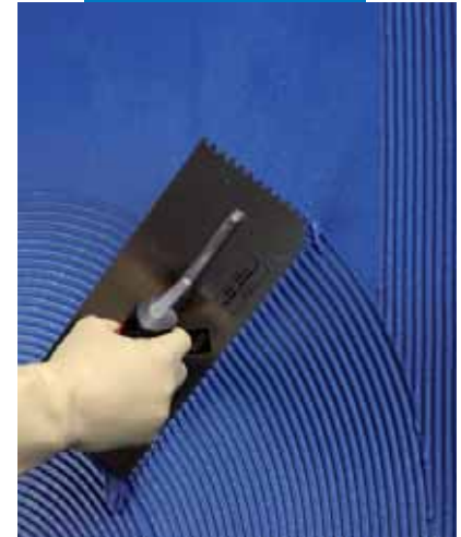
Spreading blue Kerapoxy Design used as an adhesive with notched trowel
