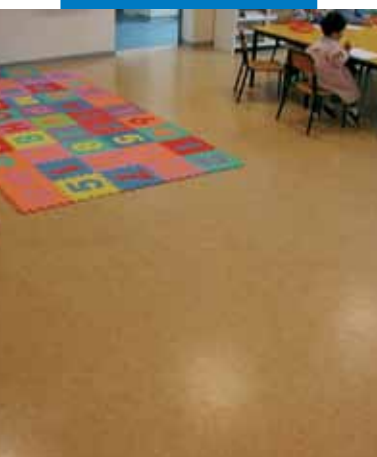
Linoleum applied on screed previously levelled with Ultraplan Eco - Mirabello kindergarten - Cantù (Como) - Italy
